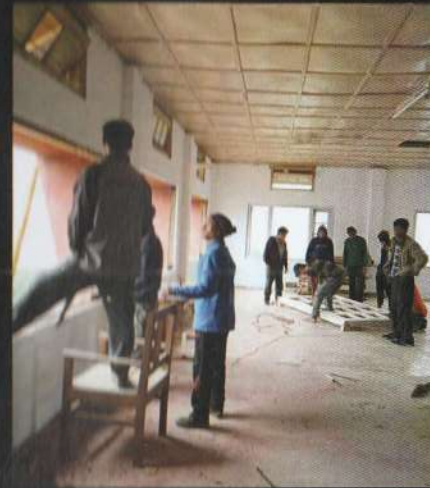
Workers renovating the Tribal Museum 2020.
